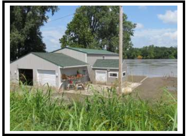
Subject Property After Flood
